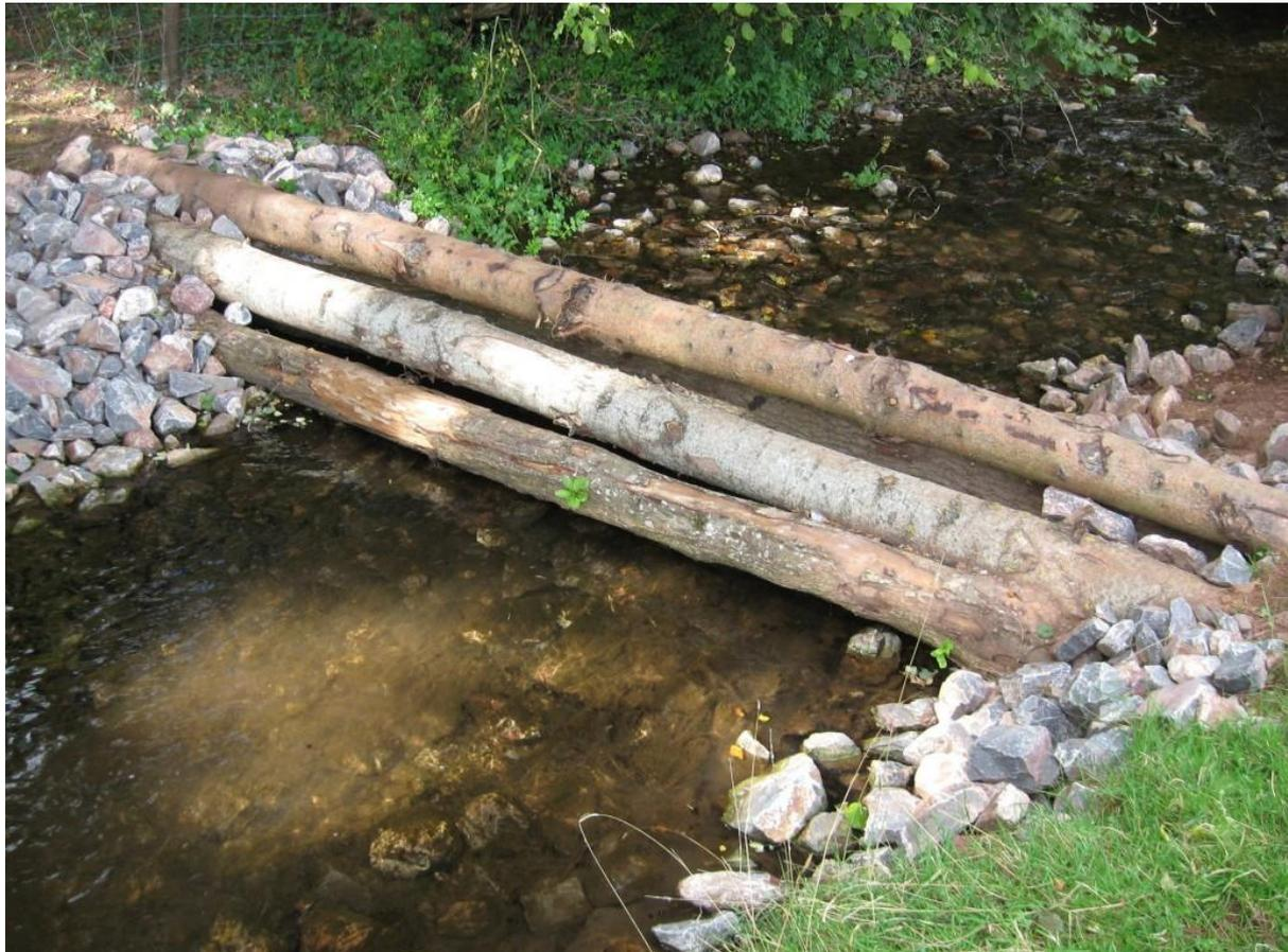
*A typical “leaky” dam or runoff attenuation feature (RAF) made from natural materials.*
